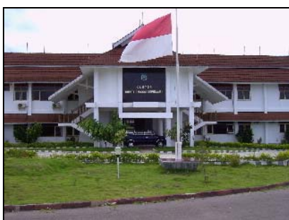
The Regency Offices
