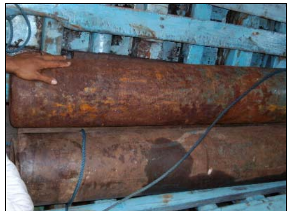
Figure 46 - Corroded Oxygen Tanks (donated by IMA in 1990s) on KM Nurul Bahari
