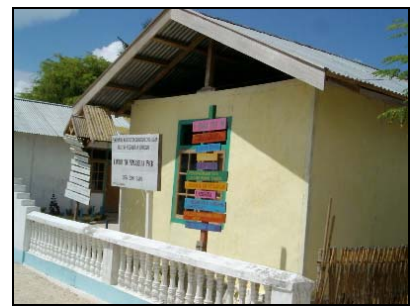
Village Offices - rebuilt by Army
