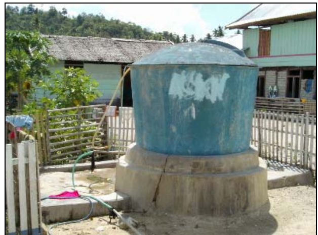
Fresh water system which often runs dry
