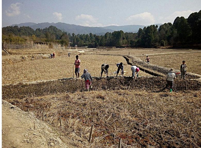
Preparation of terraces & trenches for rice fish farming.
