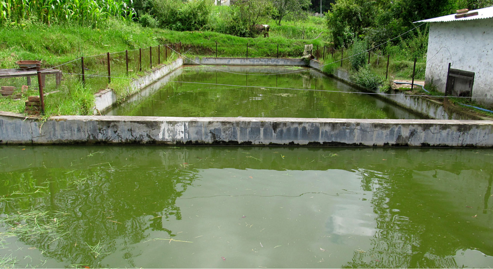
View of two cement fish tanks.
