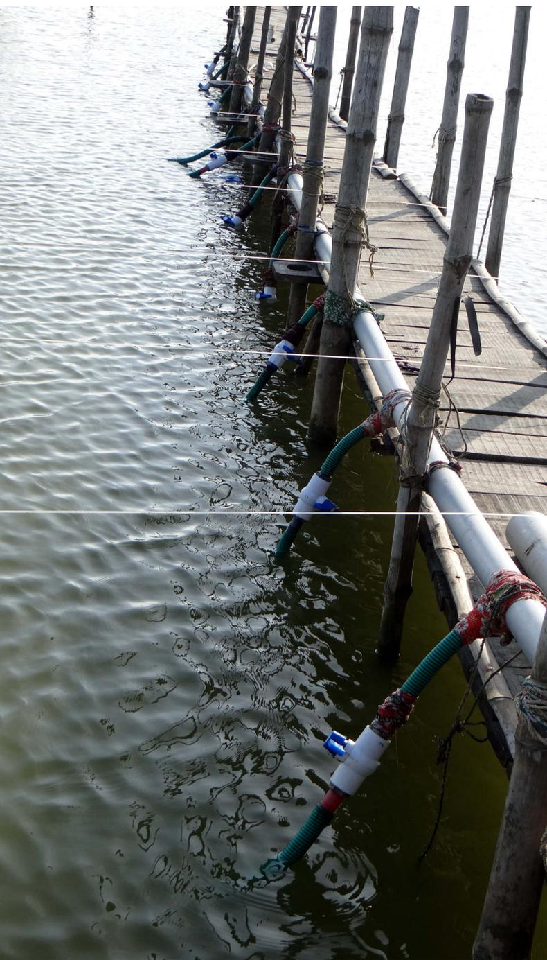
*Several units are interconnected using the main pipe from the pump.*
