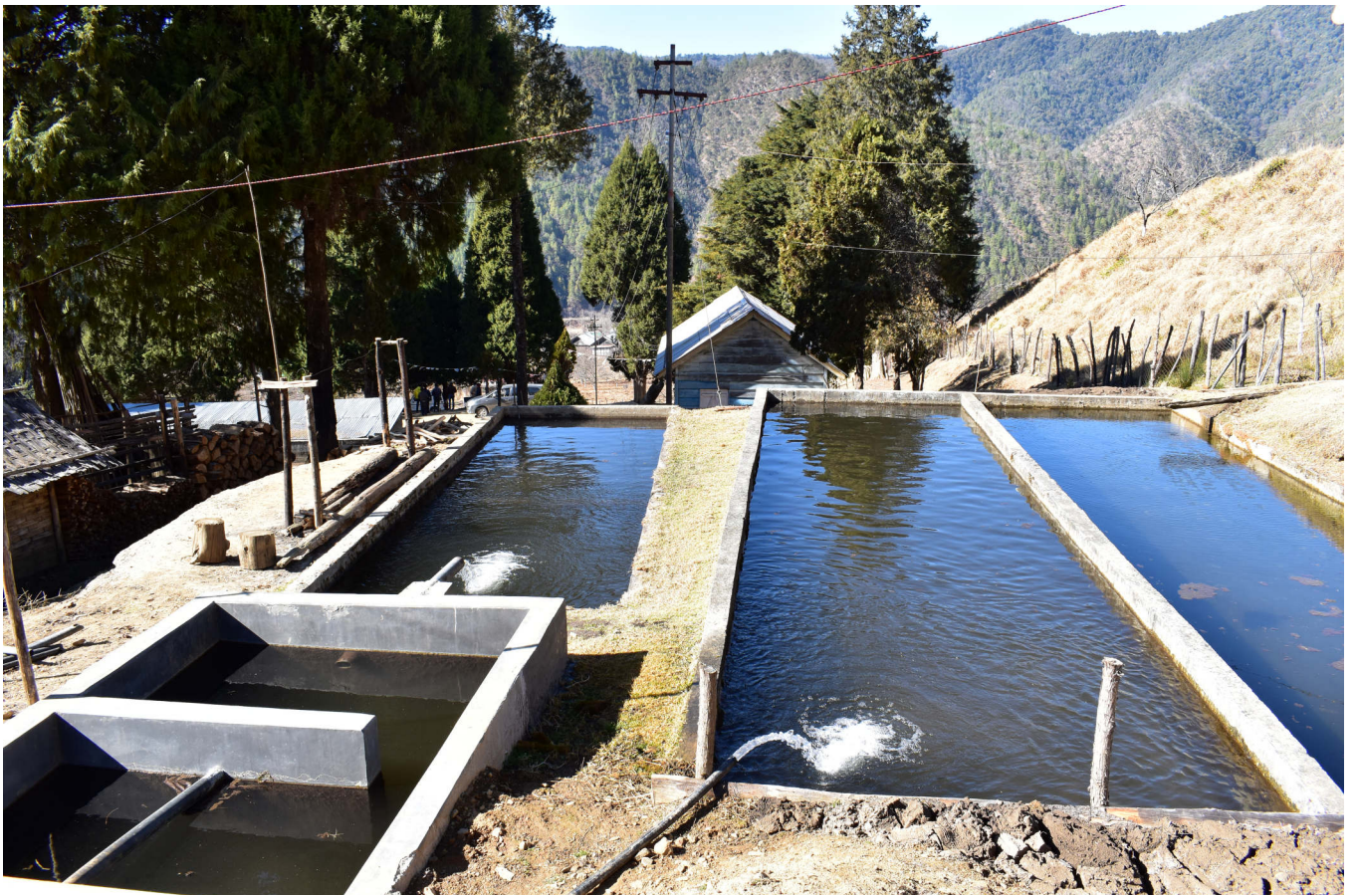
Above, below: Earthen and concrete raceways at Shergaon, West Kameng District under DoF, Arunachal Pradesh.
