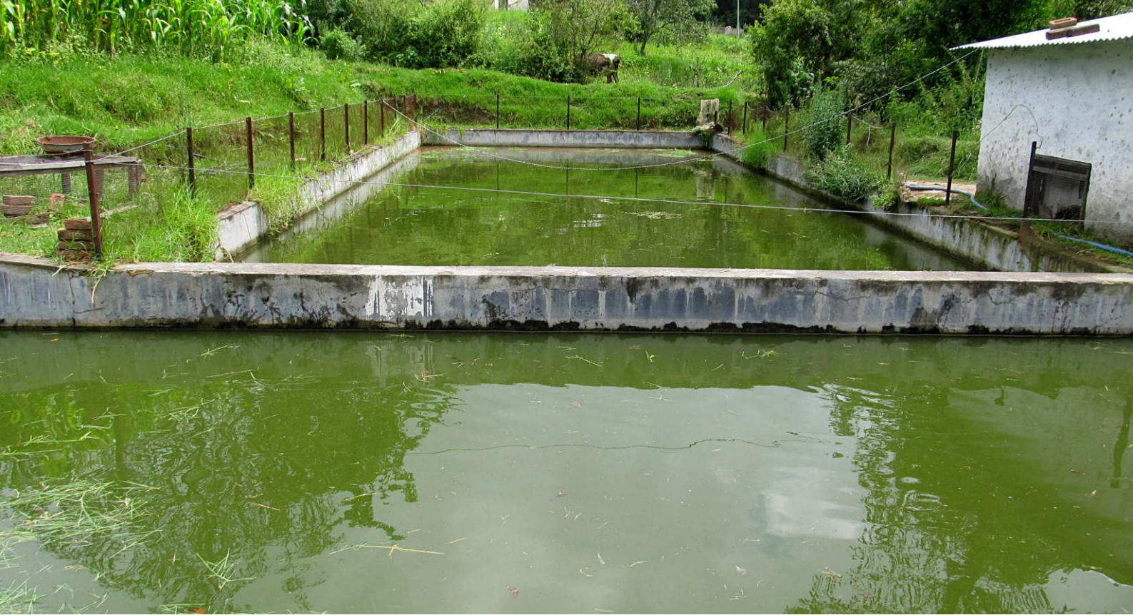
View of two cement fish tanks.
