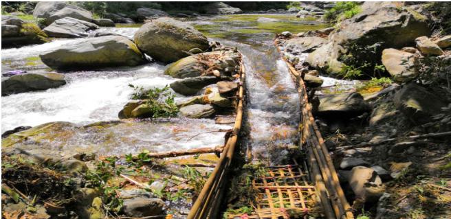
Operation of neuta over the Choskorong Kho River.
