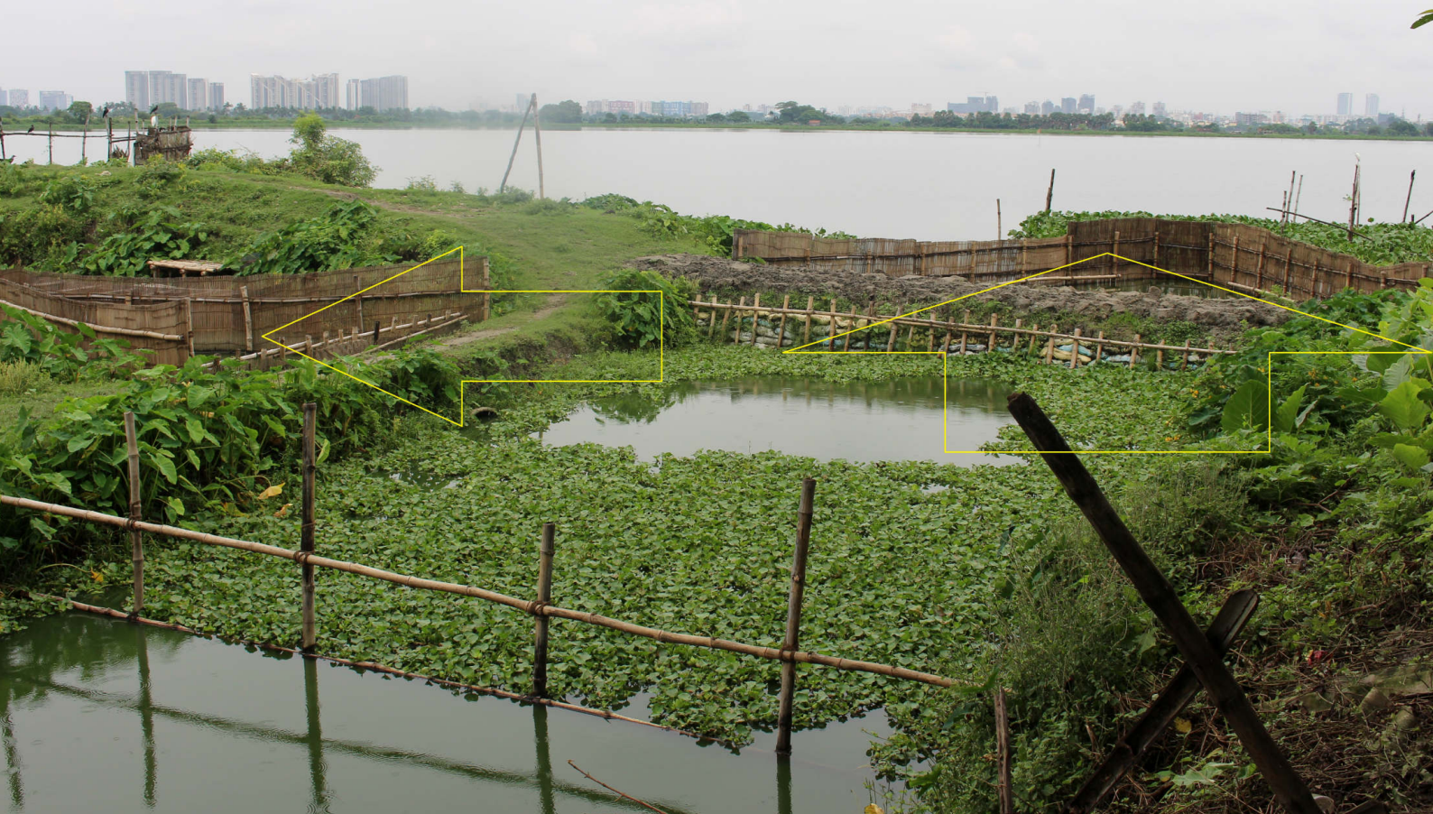
Uptake of sewage water from feeder channel into fish culture bheries through bamboo fencing.
