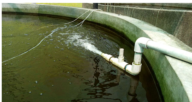
Water inlet generating circular flow in RAS cement fish tank.
