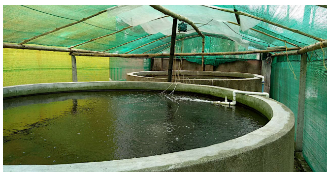
Two RAS fish tanks under shade.
