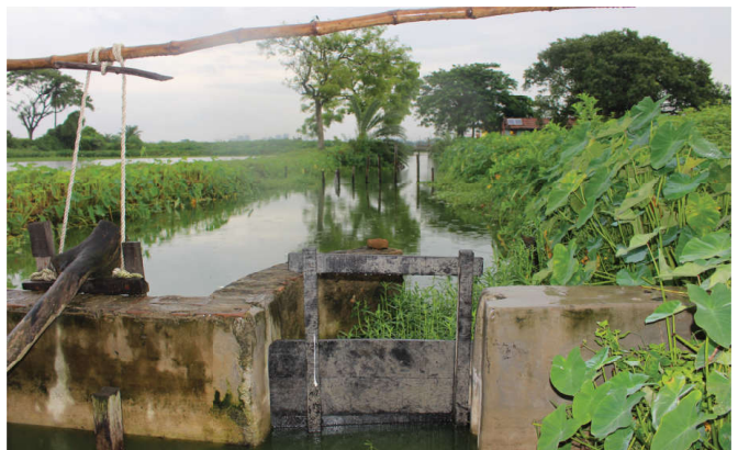
Indigenous switch-gate in the sewage feeder channel to regulate inflow to fish ponds.
