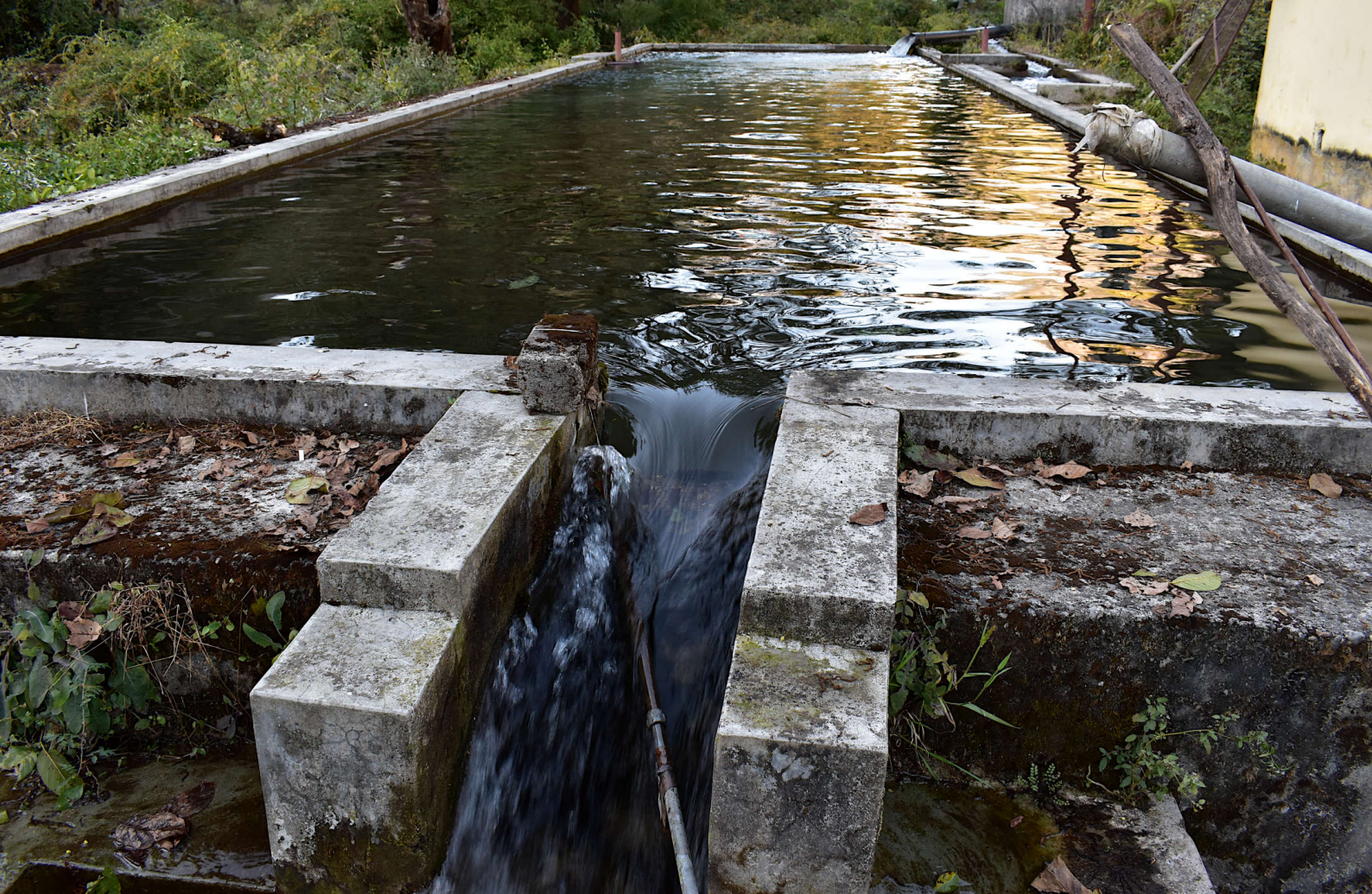
Sedimentation tanks at Bairangana.
