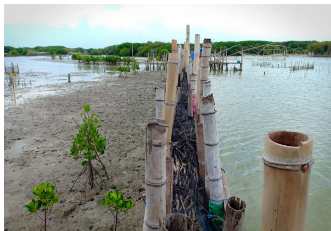
Photo 3: Permeable dams in Timbulloko (left) and Purworedjo (right), end 2019, 3-4 years after building and maintenance.
