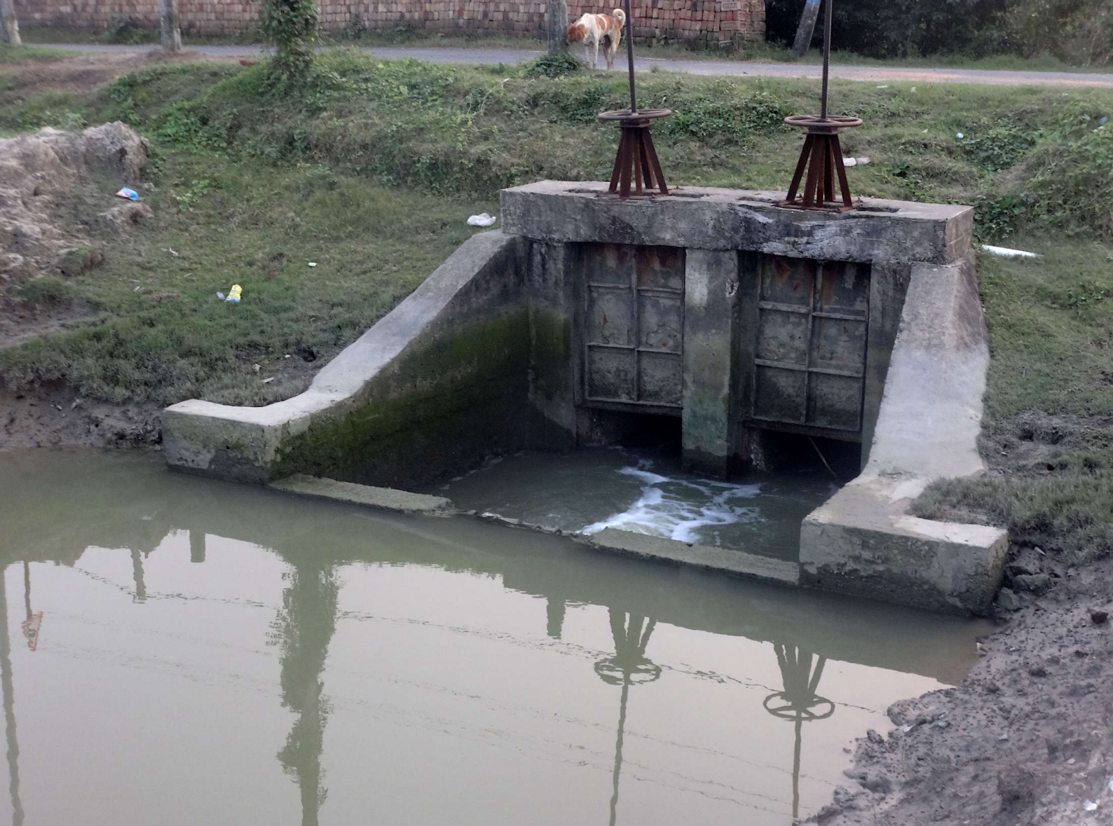
Sluice gate constructed in a canal.
