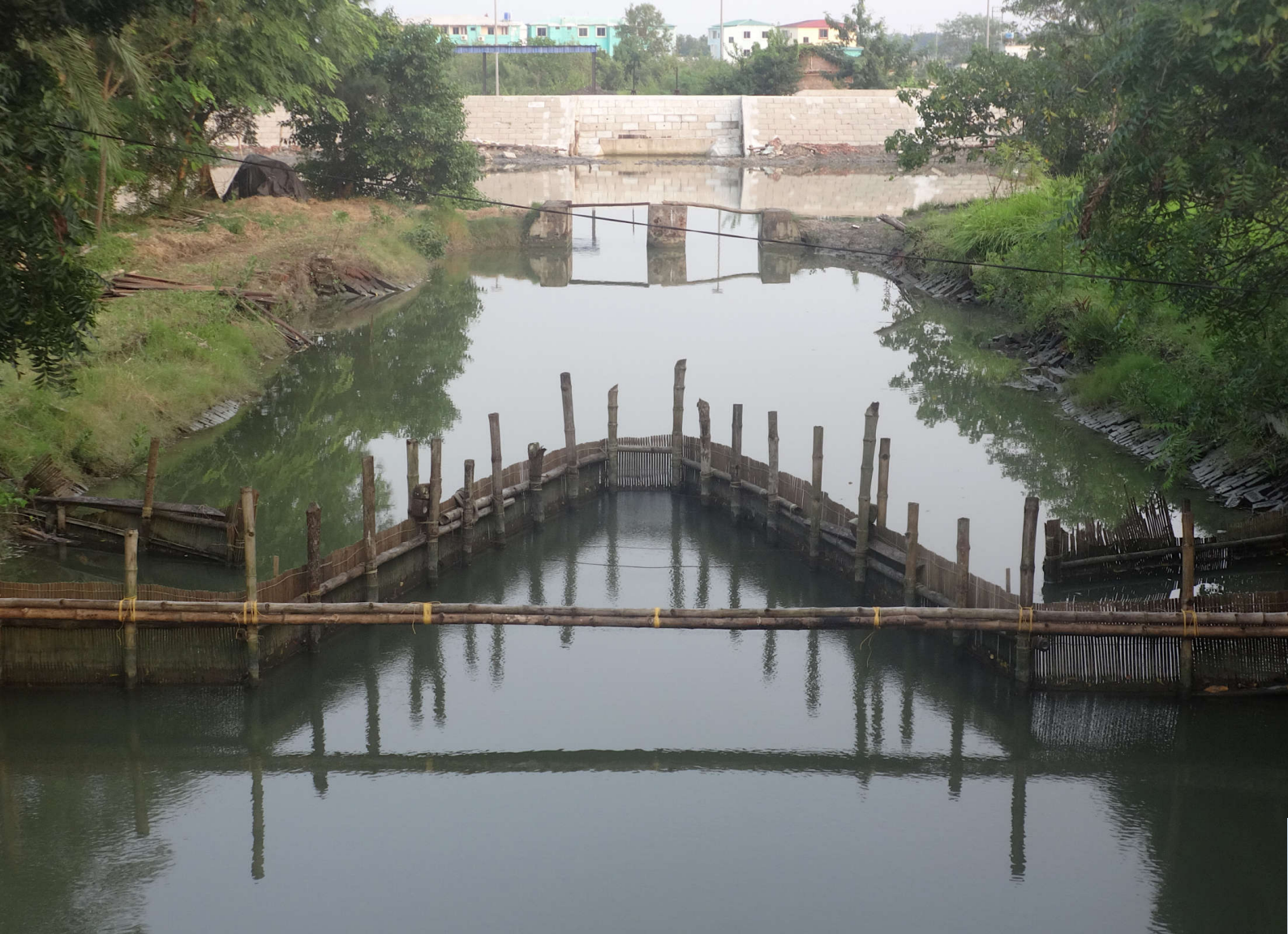
Structure for allowing entry of fish seed into large pond.
