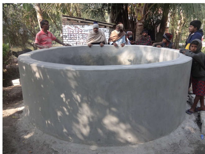
10 m tank built with state government support.
