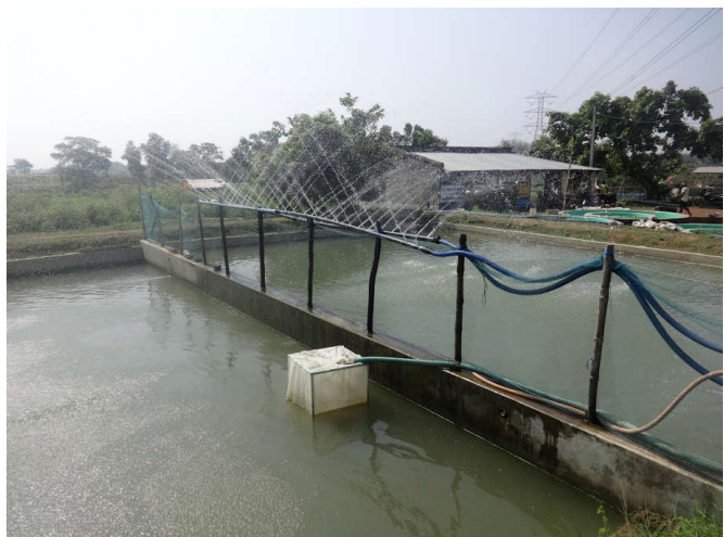
Overhead water sprinkler in fish holding pools.
