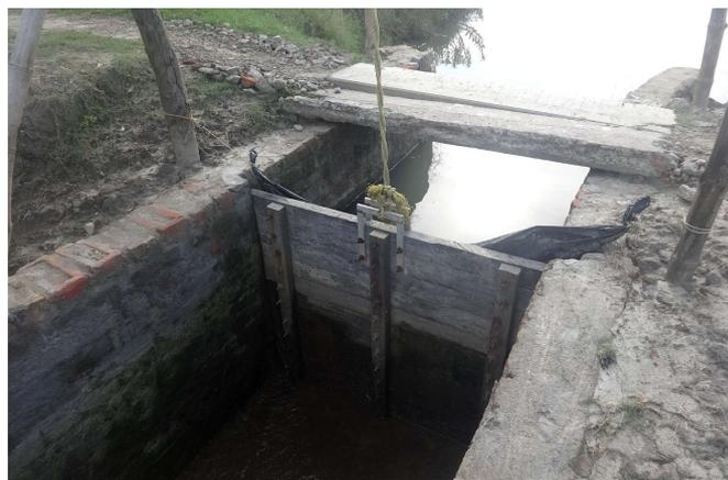
*Sluice gate or water gate with wooden shutter in a bheri.*
