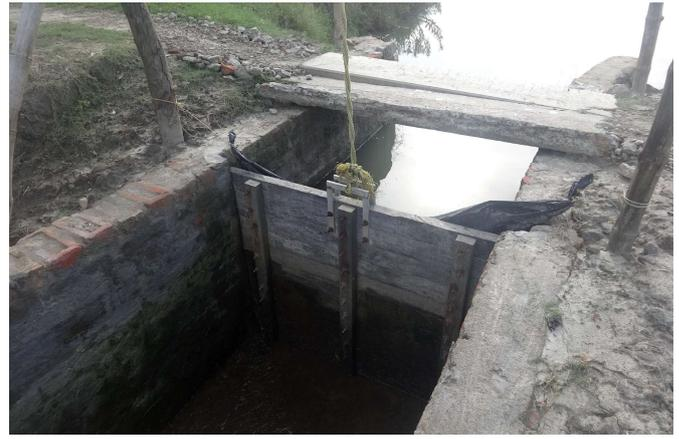
*Sluice gate or water gate with wooden shutter in a bheri.*
