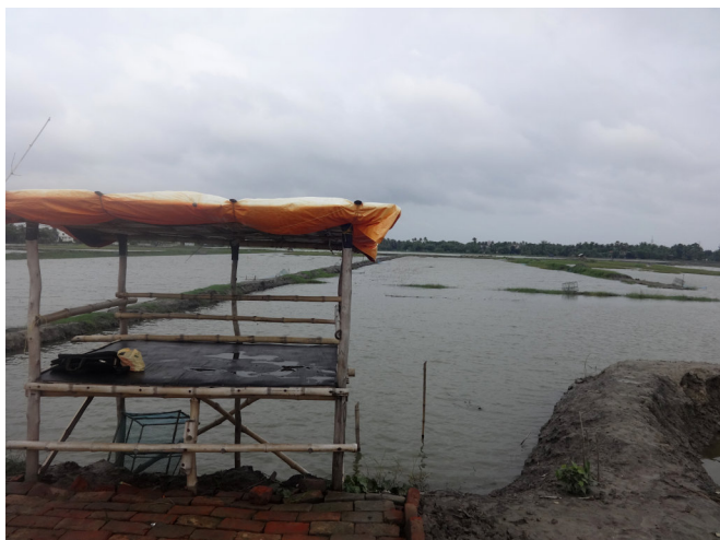
Night shelter under construction for watchman.
