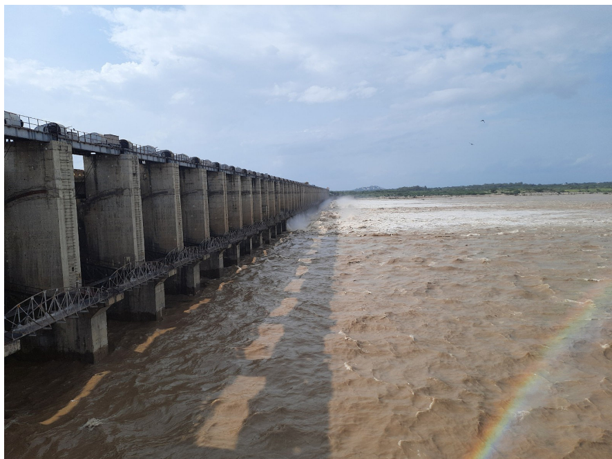
A view of Jurala dam.
