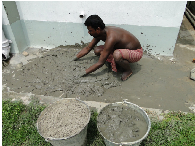
Fig. 5: Preparation of bottom with 1:1 soil and sand.
