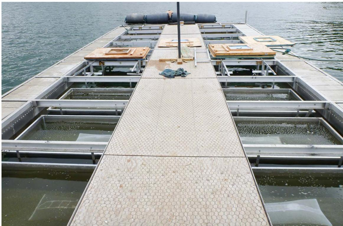
1. Bolt 25 × 25 mm aluminium angle to the top of the Flupsy frame directly above and parallel with the top of the discharge channel. They should run the entire 12 000 mm length of the channel.
