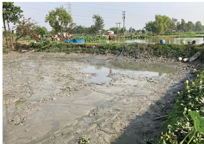
Dewatering of pond prior to scientific aquaculture.
