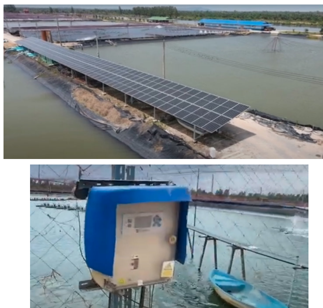
Figure 4. Using solar power system with a smart aerator control system in a closed intensive system for white shrimp farming at Kokhet Farm in Tha Chang District, Surat Thani Province.
