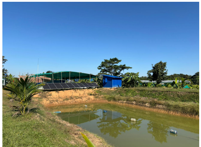
Solar panel for electricity supply.
