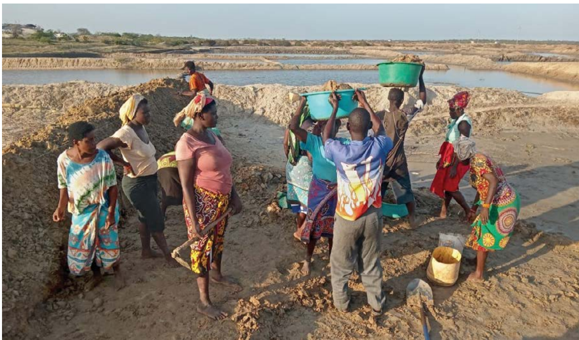
FIGURE 15. Women engaged in pond construction
