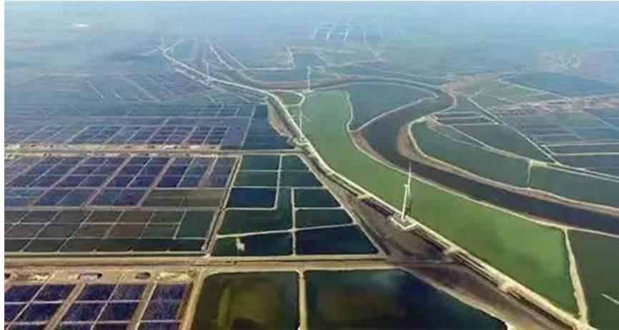
FIGURE 2. Location and overview of Bohai Bay saltworks
