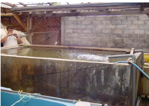
Concrete sand filter tank for a small hatchery – approximately 10 m 3 capacity.
