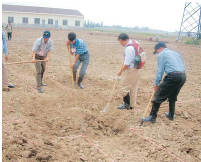
Participants in the integrated farming training course - hard at digging ditches
