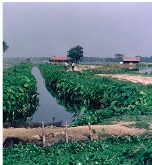
Open channel through which sewage is flown. Lush growth of Colocasia seen on either side of the channel.
