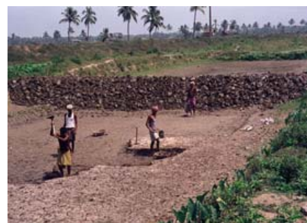
Silt is removed at least once in three years.
