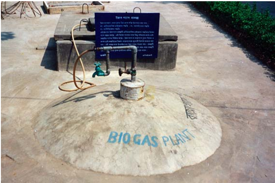
Efficient recycling: Poultry, cattle and kitchen waste is passed through a biogas digester to produce energy, then the residual slurry is used to fertilize ponds, boosting fish production
