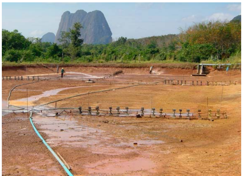
Figure 2: Removal of SPW by pressurised pumps is becoming less common
