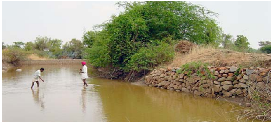
A check dam in India. Courtesy Murray and Little
