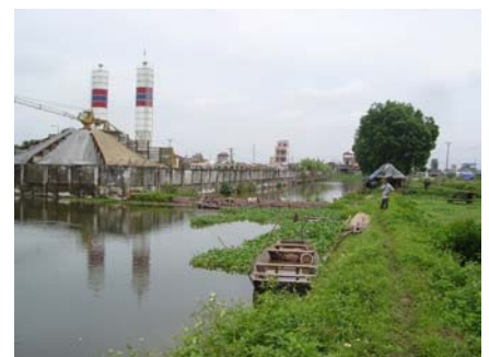
Construction material yard built on a former fishpond.
