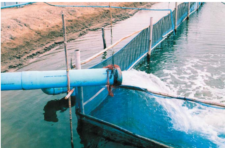
Close up of seawater inlet and containment fence.
