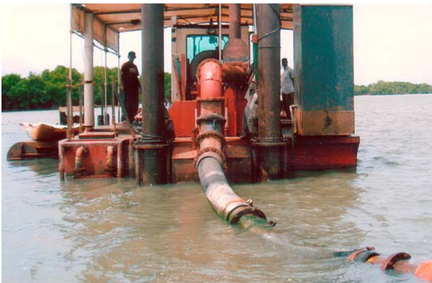
Pumping sediment from the Dutch canal.
