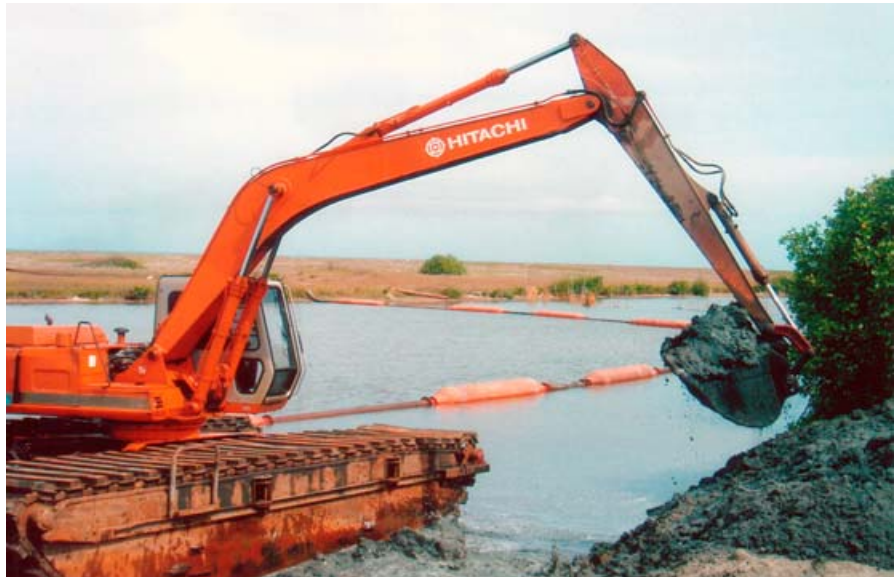
Maintenance of the Dutch Canal - years of accumulated silt must be removed.
