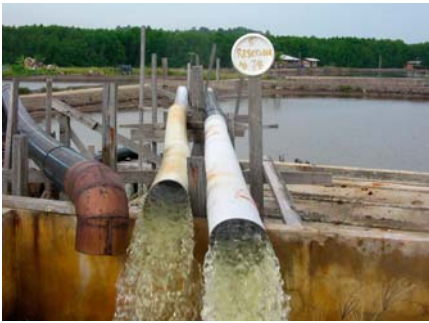
Pumping water to reservoir pond.
