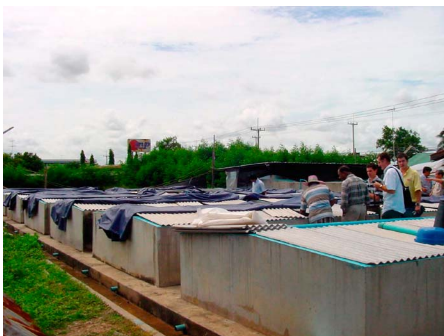
Concrete tanks for nursing PL.
