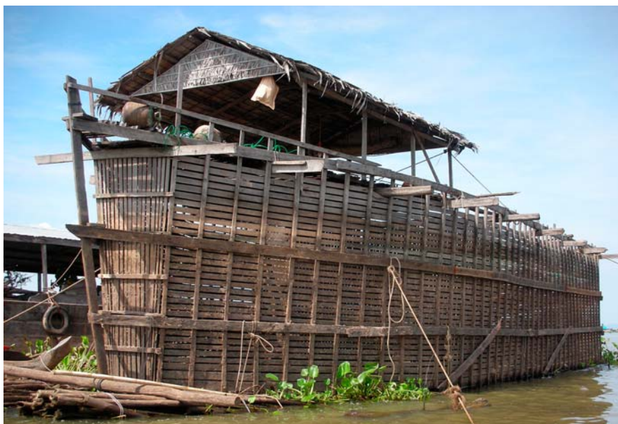
Constructing a cage for silver striped catfish at Chnok Trou on the Great Lake, 2006.
