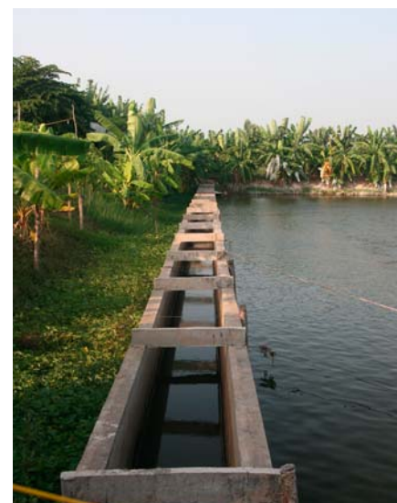
Raceway inlet for water from the river.
