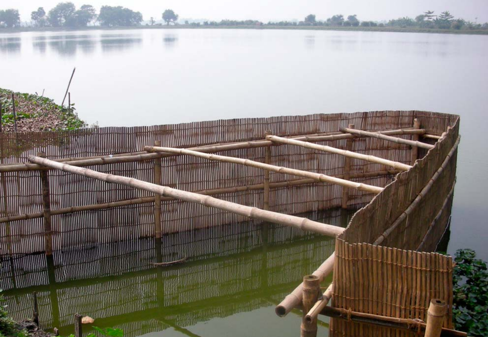
A pond drainage outlet.
