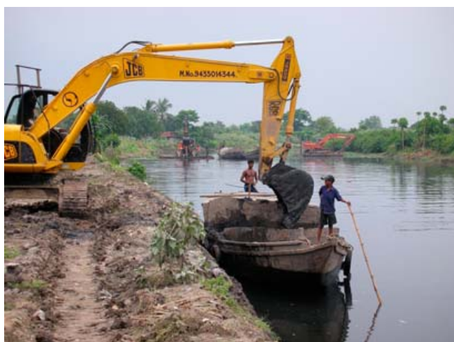
Dredging the main sewage canal above Bantala.
