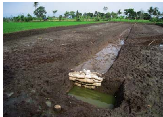
Harvesting sump in a newly constructed nursing pond in a former rice field, Cianjur.
