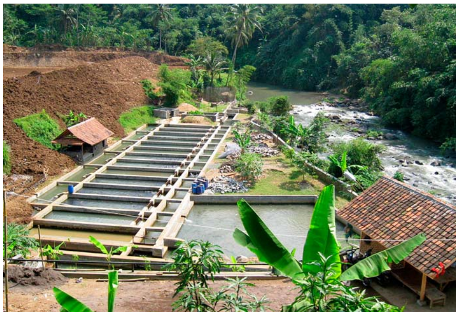
A newly constructed running water pond farm in Subang.
