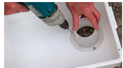
Attaching a K Box Cone to a tub with a 92 mm diameter hole cut in its base.
