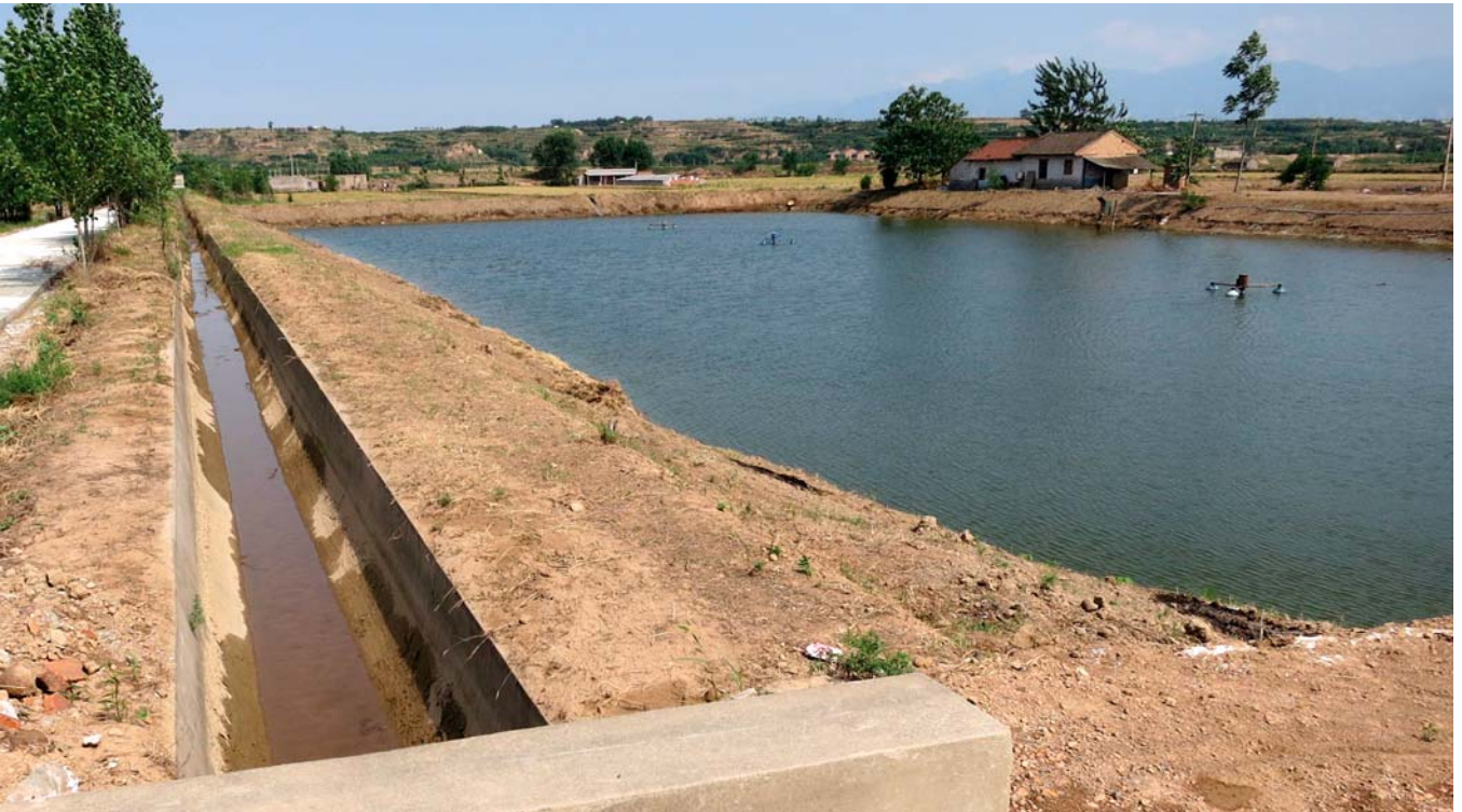
Renovated pond and water supply at Yunyang small-scale farmers cooperative in Shanxi Province.
