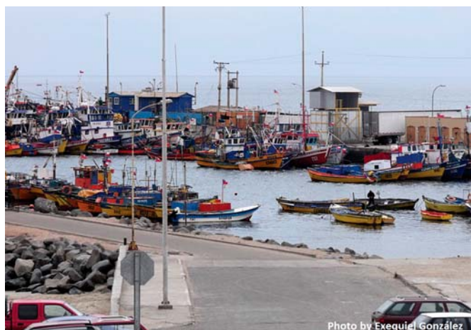
Port of Caldera.
