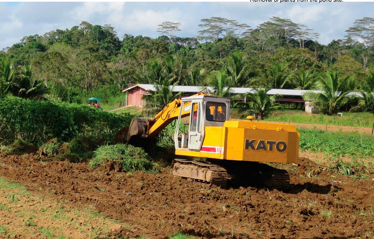
Removal of plants from the pond site.
