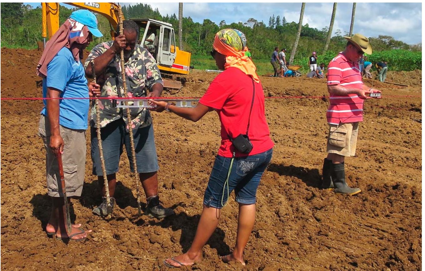
Measuring the level of the future pond bottom with spirit levels.
