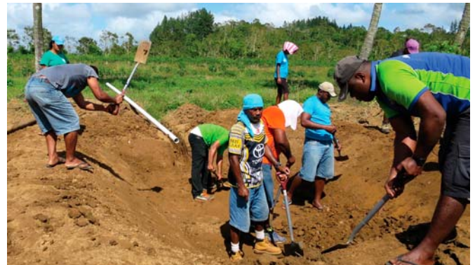
Shaping and compacting the dikes and laying drainage pipe.
