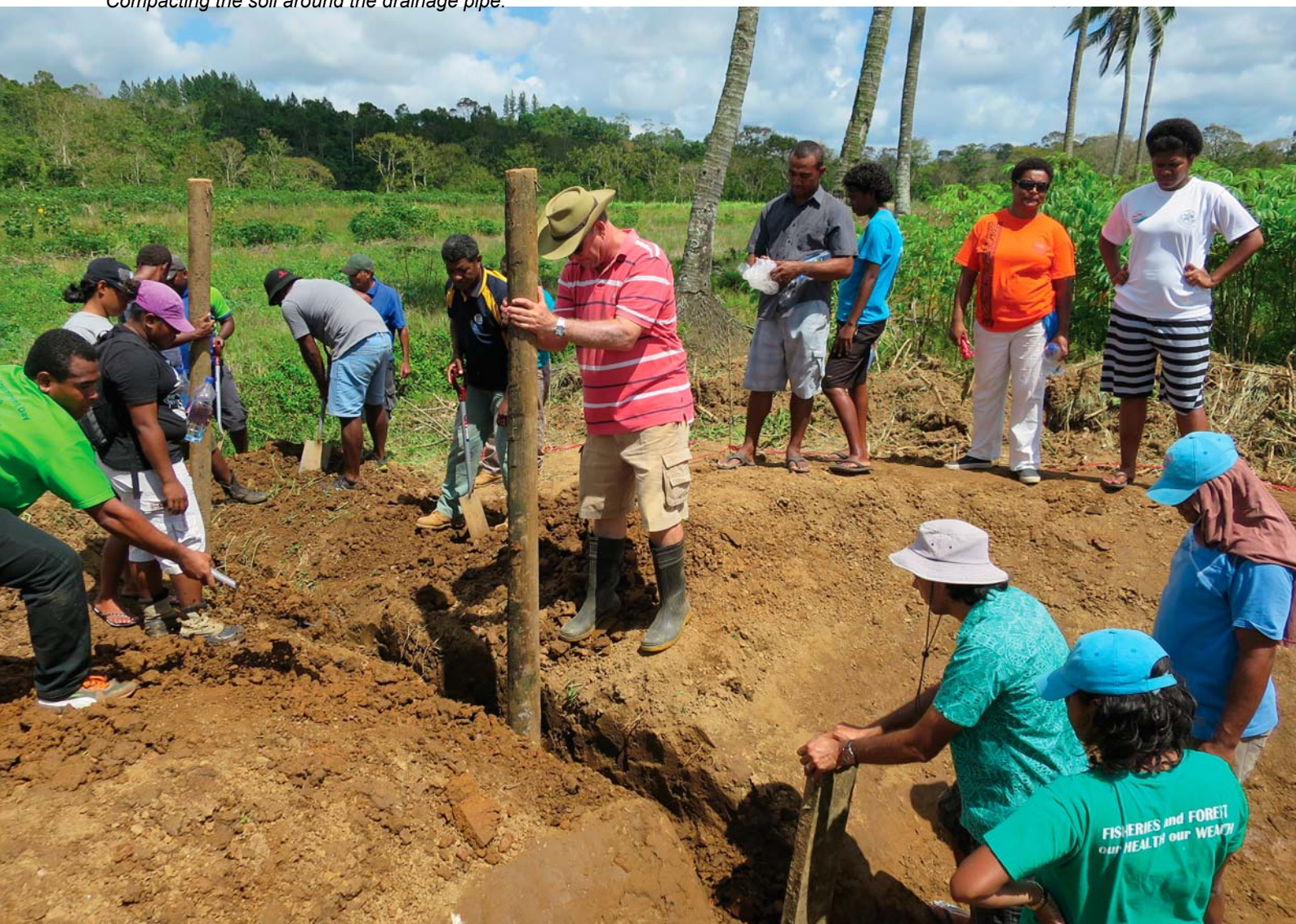
Shaping and compacting the dikes and laying drainage pipe.
