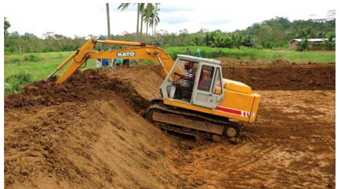
Excavating through the dike to place the drainage pipe.
