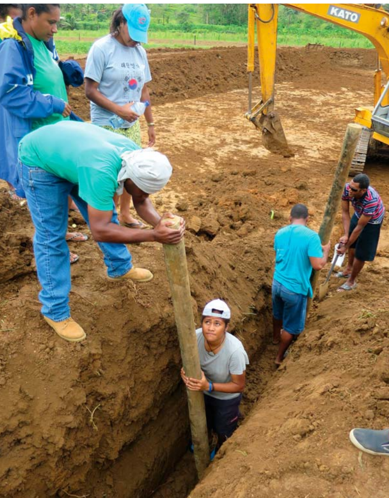
Compacting the soil around the drainage pipe.
