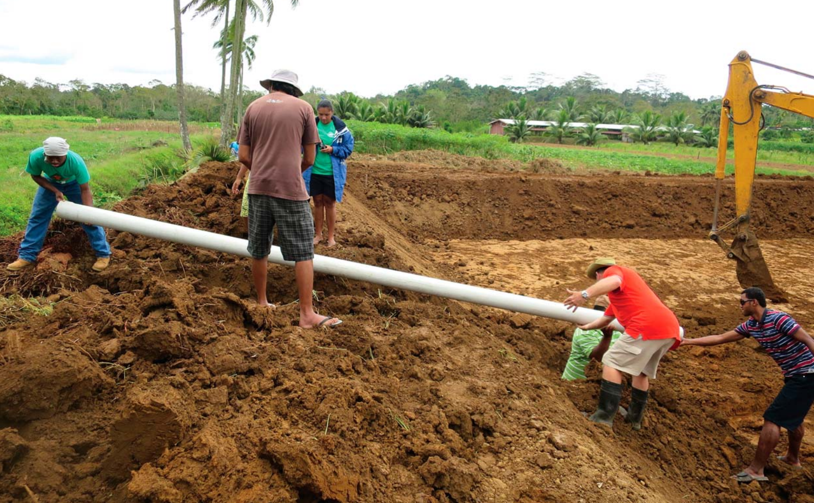
Placing the pond drainage pipe.
