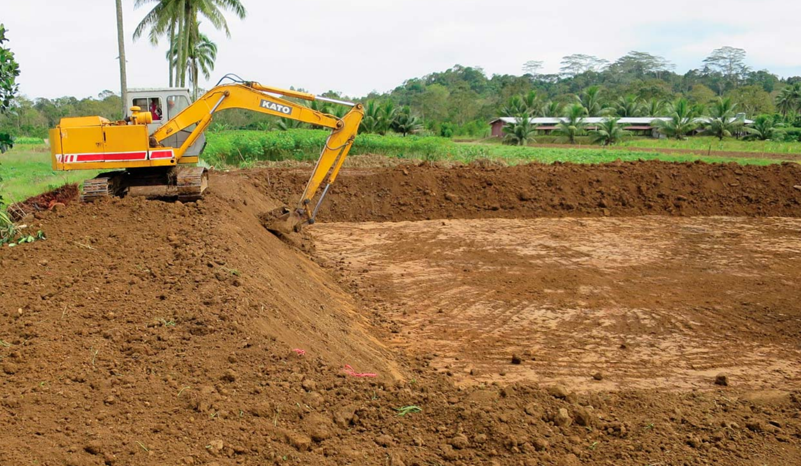
Shaping the slope of a dike.
