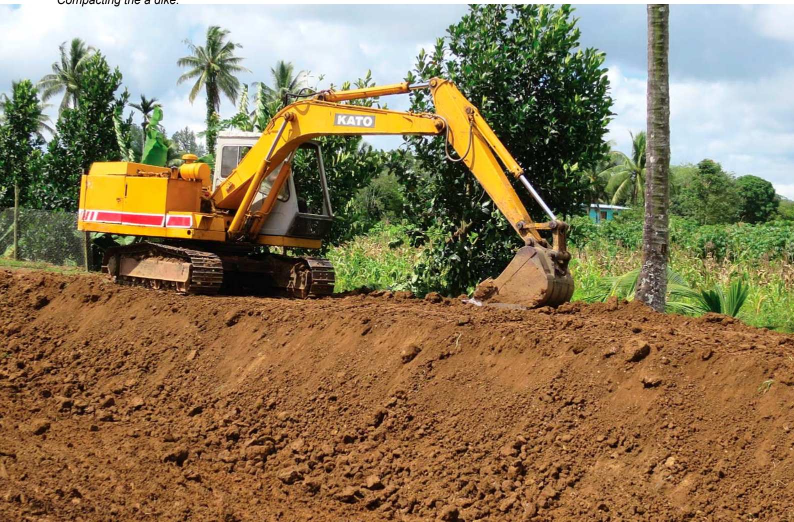
Compacting the a dike.
