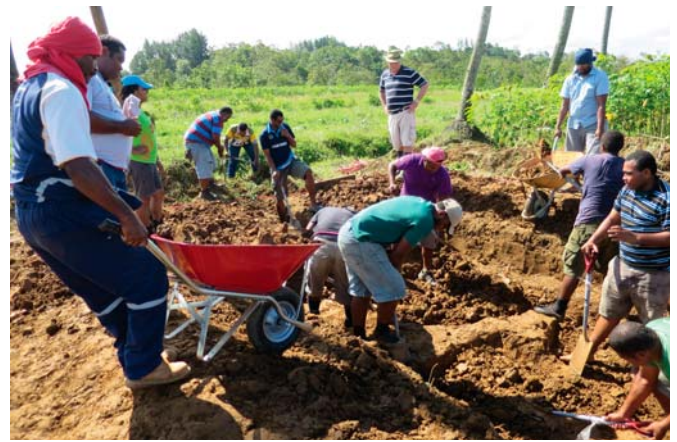
Doing it the hard way: Manually digging a small pond.
