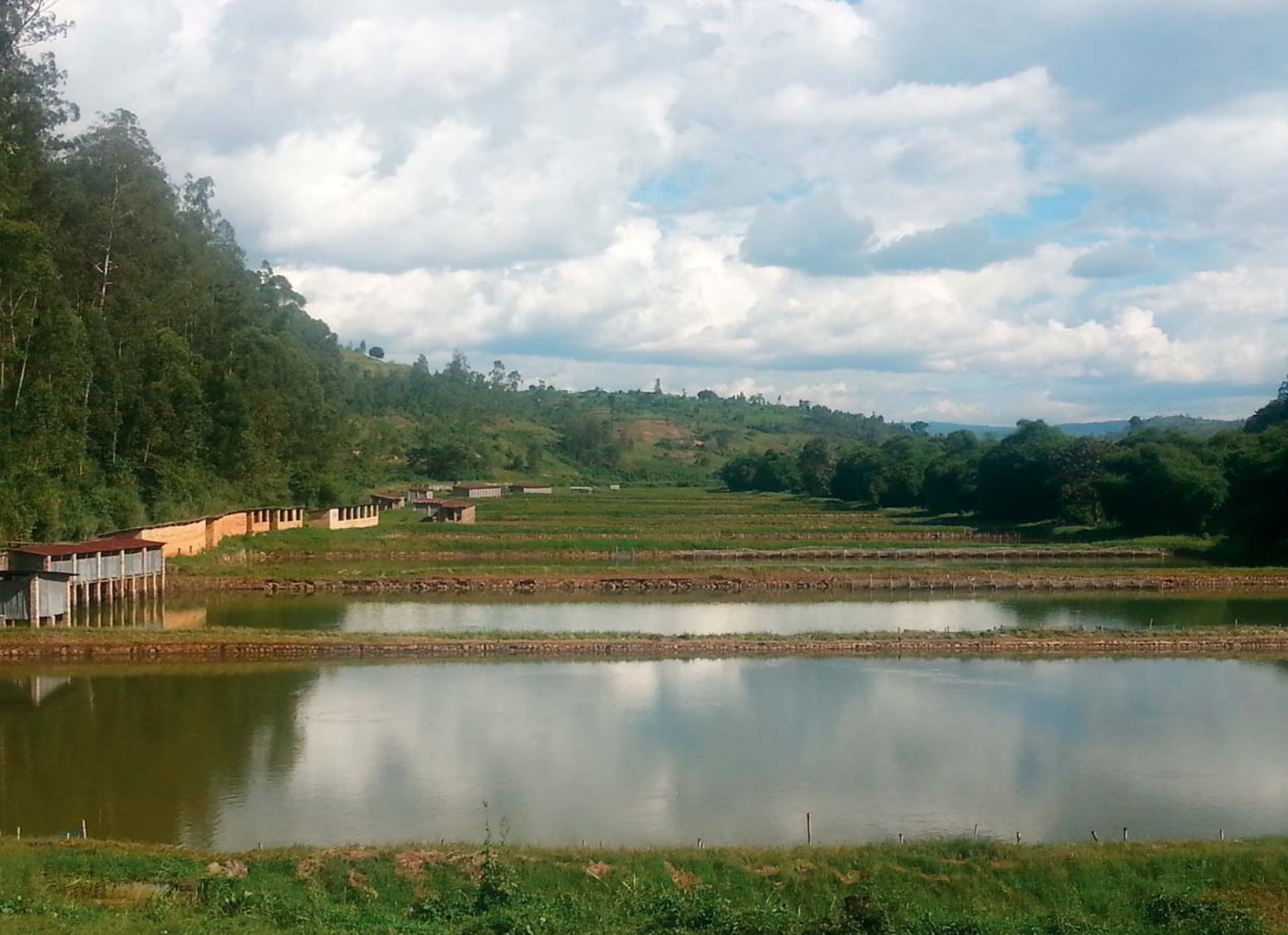
General view of Kigembe Fish Centre.
