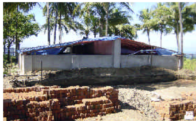
Shrimp hatchery under construction in Rakhine State
