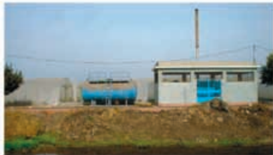
Water boiler in a tilapia hatchery in Egypt
