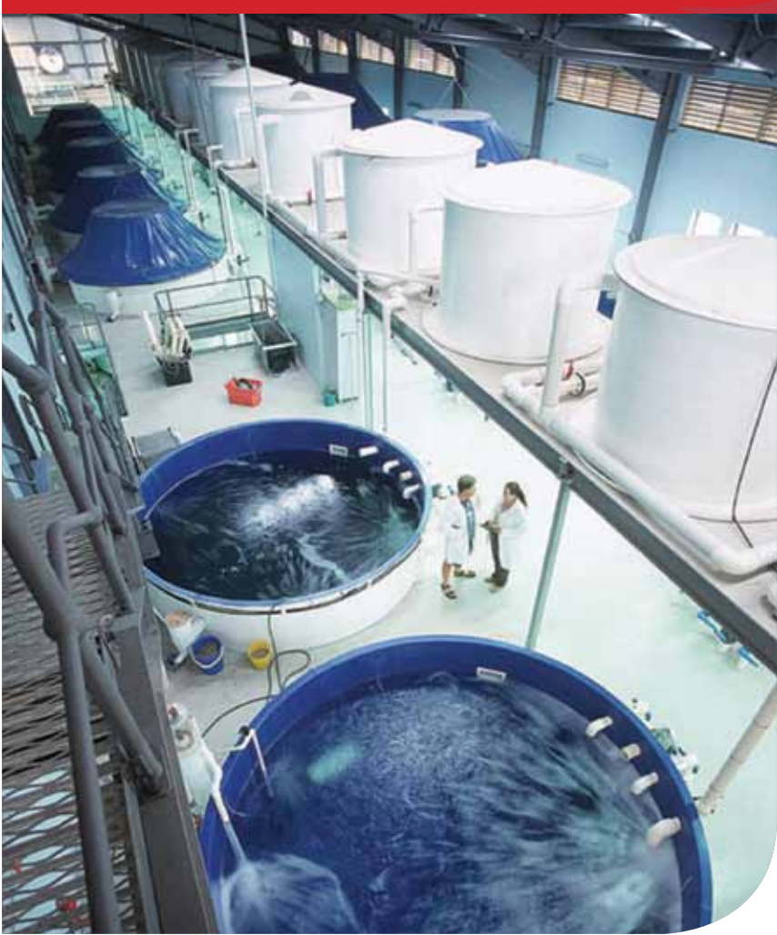
Figure 9 Fibreglass tanks used for holding tiger grouper broodstock at the Northern Fisheries Centre, Cairns, Queensland, Australia. The tanks in the foreground are about 20 m 3 in volume and each is fitted with a recirculation system comprising a biological filter (white elevated tanks) and ozone system to maintain water quality, and a heat exchanger to maintain water temperature. Some tanks are covered (background) and fitted with computer-controlled lighting systems to control day length as well as water temperature. (Photo: Queensland Department of Primary Industries and Fisheries)
