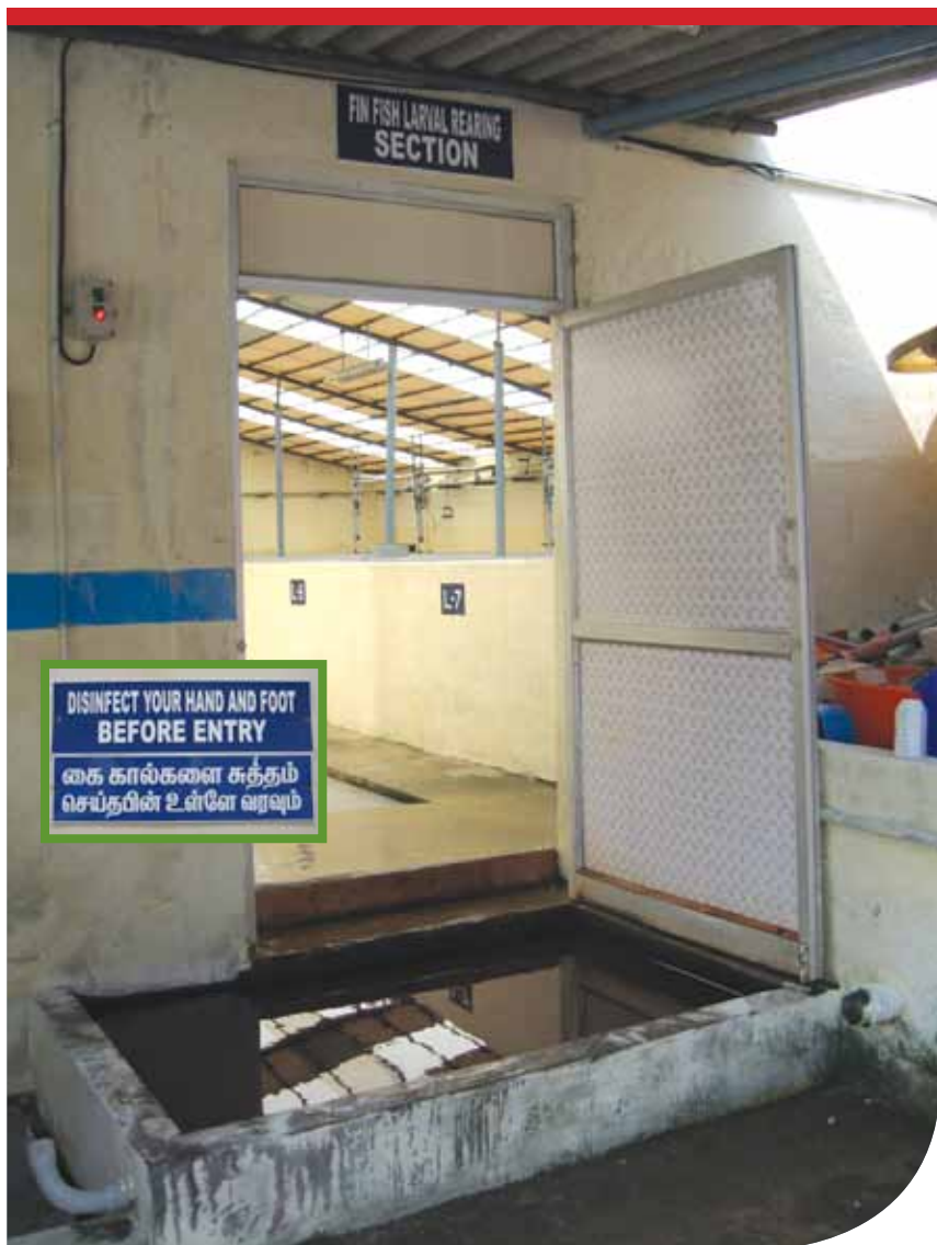
Figure 6 To ensure biosecurity, hatcheries should be fitted with lockable doors and each entrance should have a footbath. Signage should include instructions to disinfect hands and footwear on entry (inset) and note restriction of unauthorised visitors (not shown). (Photo: M. Rimmer)
