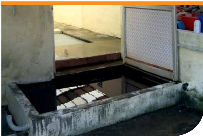
Figure 5 Access doors to nursery facilities should be fitted with a footbath and handwash—this footbath has been designed to prevent staff or visitors stepping over or around it (Photo: M. Rimmer)
