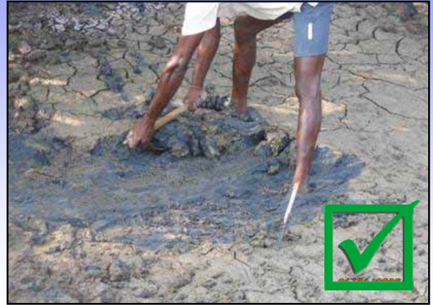
Proper removal of black soil
