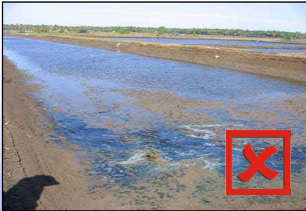
Water not proper dry
