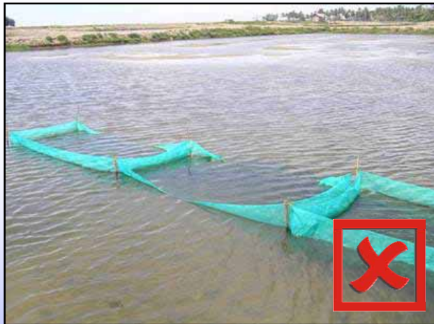
Improperly fixed hapa
