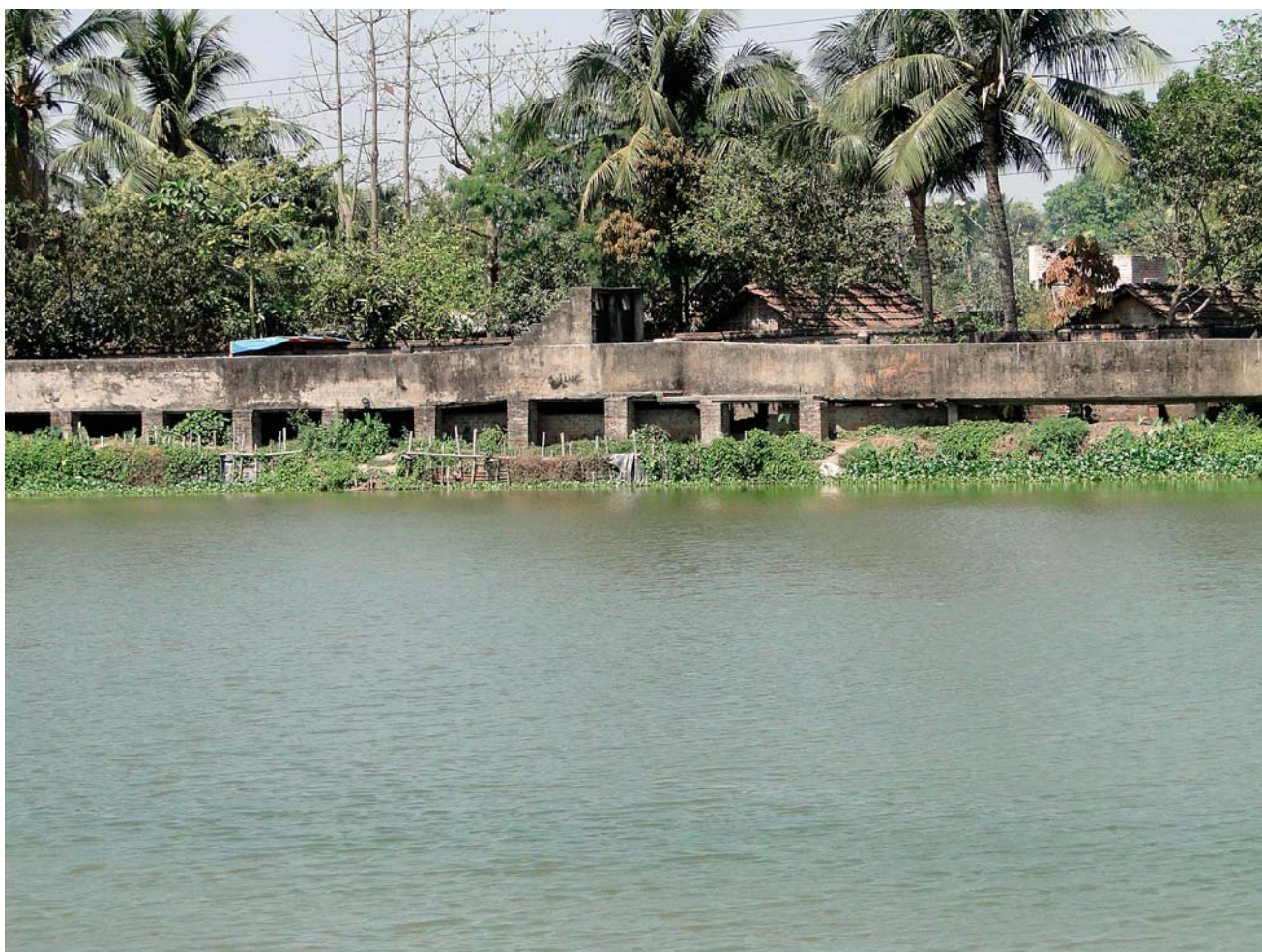
Sewage transport channel.
