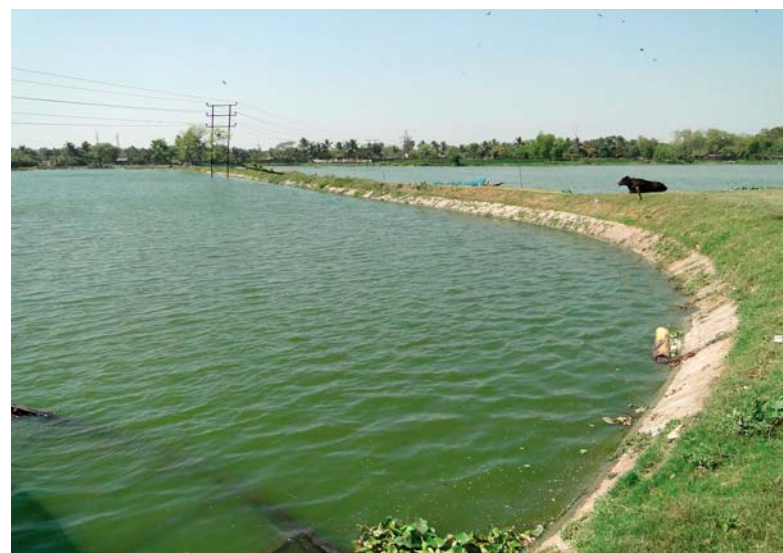
Cement lining around the edge of pond dyke.
