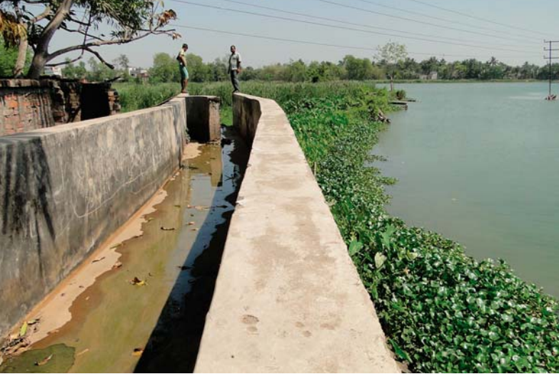
A view of sewage inlet.
