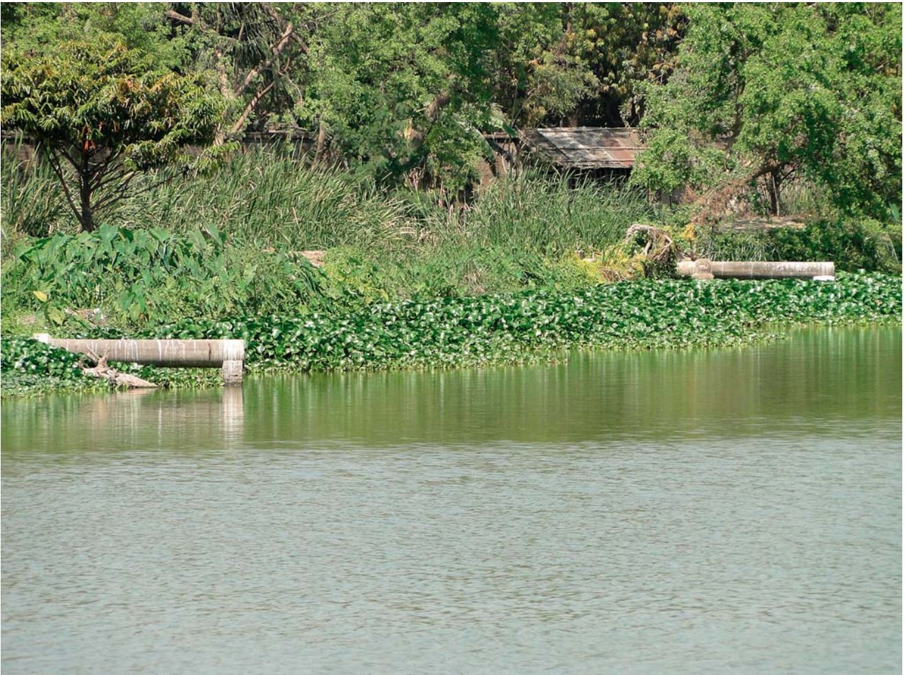
Sewage mixing water body via sewage pipe.
