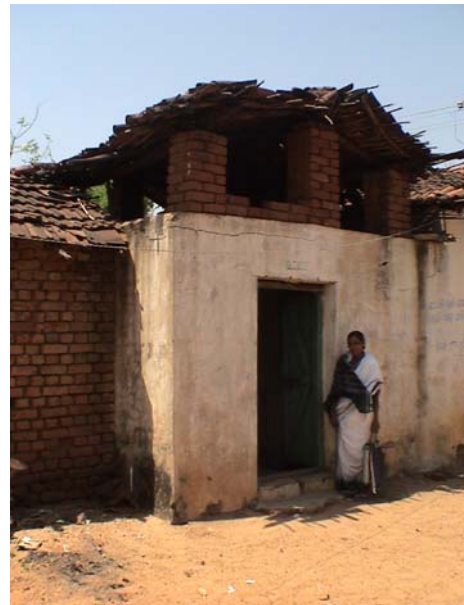
A One-stop Aqua Shop for Kandhkelgaon
