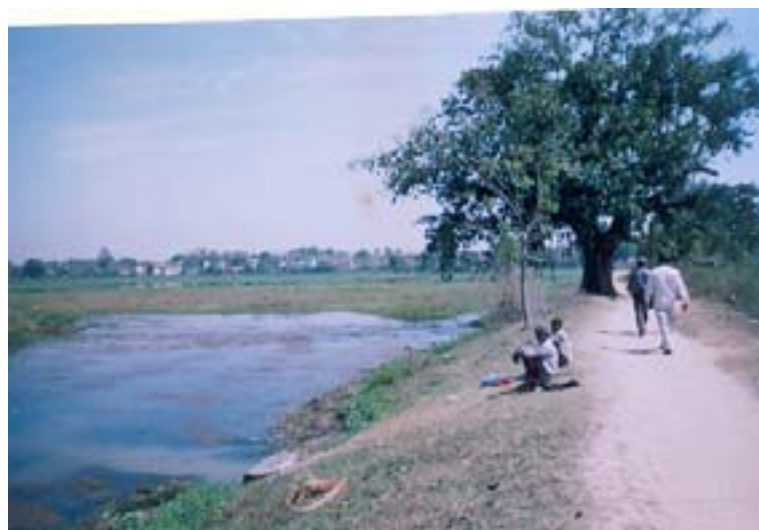
Bundu Bara Bandh – cleaning in process
