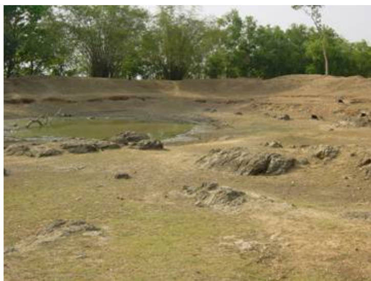
Huchak Guria in Jabarra Village, being dewatered for deepening and improvement
